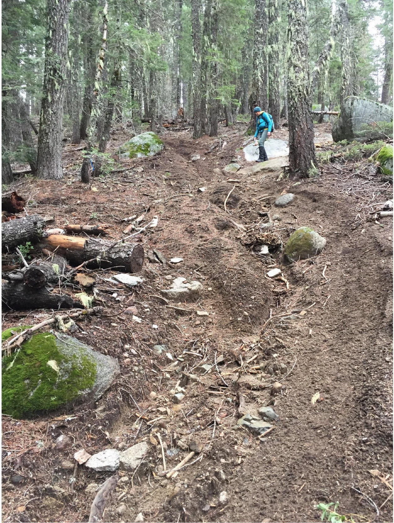
Erosion resulting from OHV use on 6M46 north of the Little North Fork of the Middle Fork Feather River.
